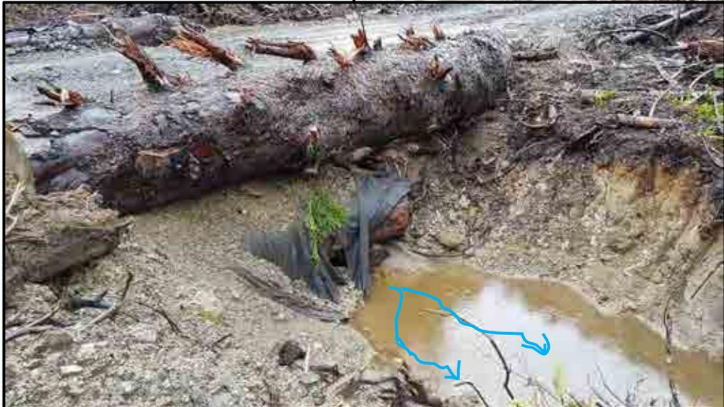
Photo 3: View of Stream 1 and stringer log bridge. Bridge to be removed and replaced. 6" flow clearance
